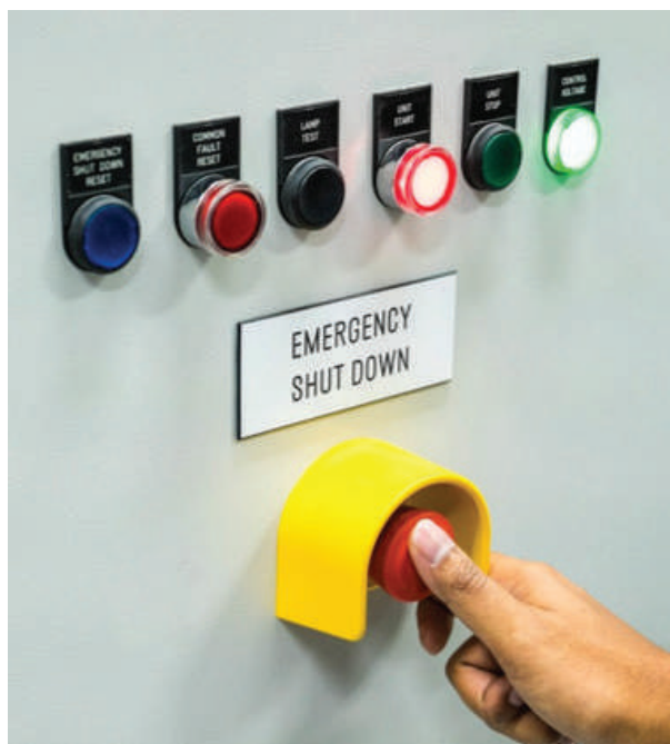
Fig. 6.1.41: Emergency shutdown system
