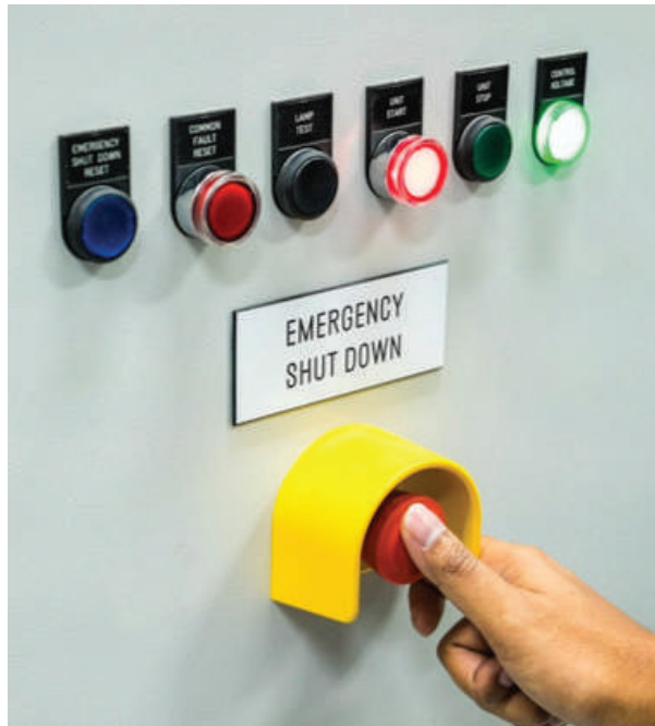
Fig. 8.1.41: Emergency shutdown system
