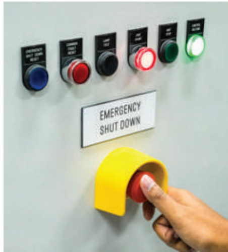
Fig. 7.1.29: Emergency shutdown system
