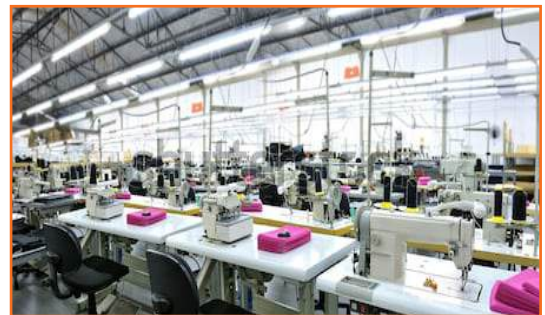
Fig.5.1.8: Use of daylight
